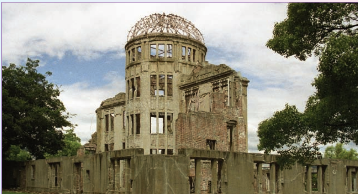
The A-bomb Dome is the ruins of the former Prefectural Industrial Promotion Hall destroyed by the the world's first A-bomb on August 6, 1945. Hiroshima Japan
